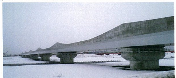
写真-7 姫川橋梁
