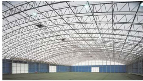
Figure-2 Photo of inside view of tent structure (Width 50m)
