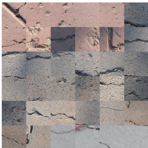
Figure 2: Input images of SDNET pavement crack
