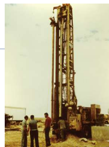
1978 Water Resources Development Project in Benghazi (Libya)
