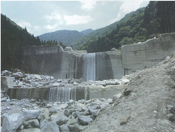
写真-8 梨子沢砂防堰堤全景 Photo 8 Nashizawa sabo dam
