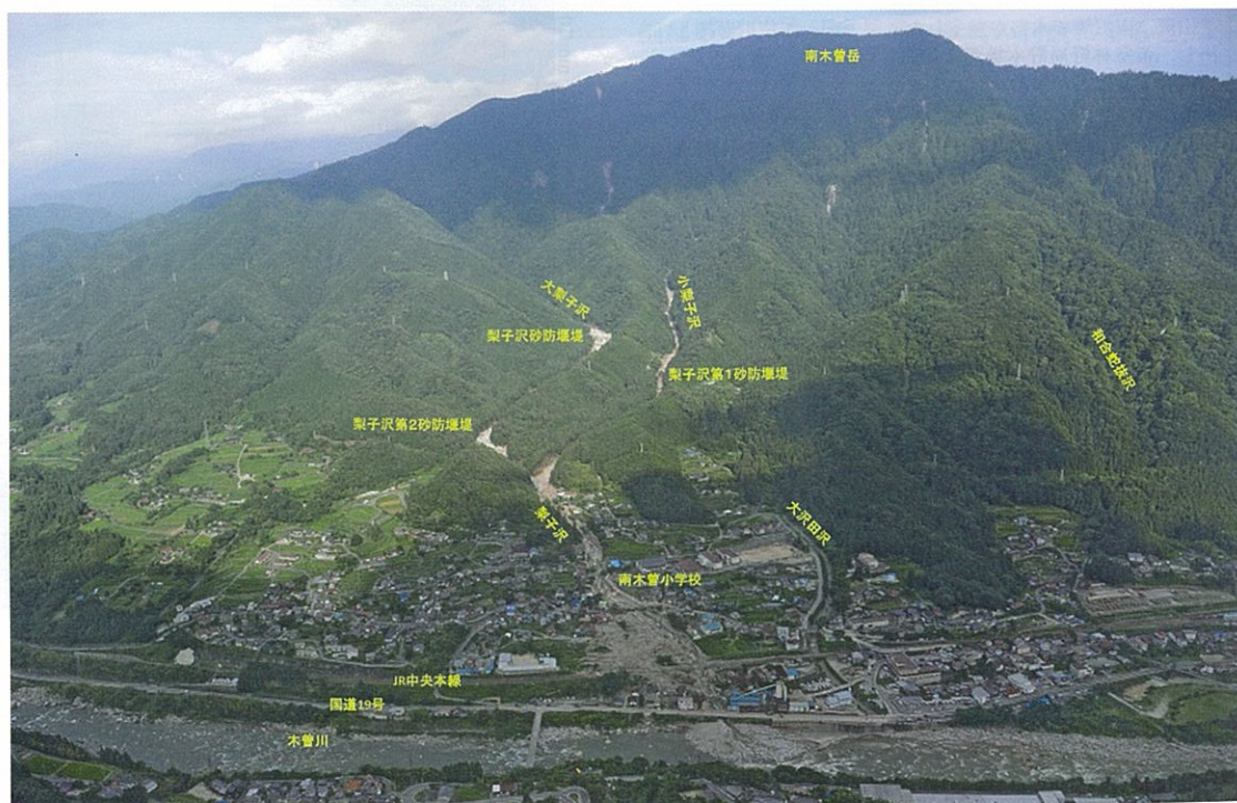
写真-1 梨子沢流域全景 Photo 1 Aerial view of Nashizawa watershed
