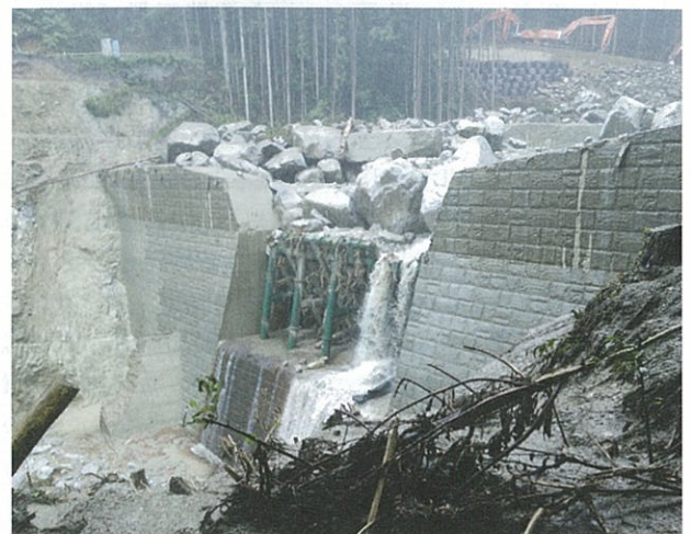
写真-10 梨子沢第 2 砂防堰堤 Photo 10 Nashizawa dai-ni sabo dam
