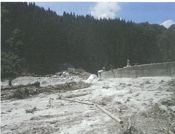
写真-9 梨子沢砂防堰堤の堆砂状況 Photo 9 Sedimentation in Nashizawa sabo dam
