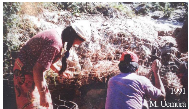
Fig. 6 Local people repairing gabions, Nepal
