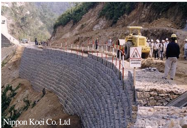
Fig. 5 Retaining wall constructed with gabion Sindhuli Road, Nepal
