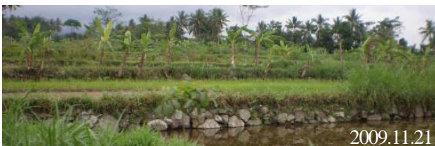
Fig. 7 Stone piling work seen at paddy fields on the hill side of Mt. Merapi, Indonesia
