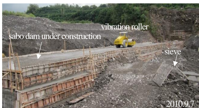
Fig. 4 Compacting of soil cement at sabo dam construction Merapi Project
