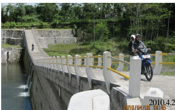
Fig. 1 Multi-purpose sabo dam used also as a bridge Merapi Project
