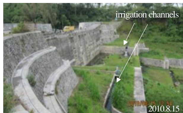
Fig. 2 Multi-purpose sabo dam used as a bridge and an irrigation water intake, Merapi Project
