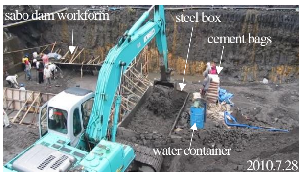
Fig. 3 Soil cement production, Merapi Project
