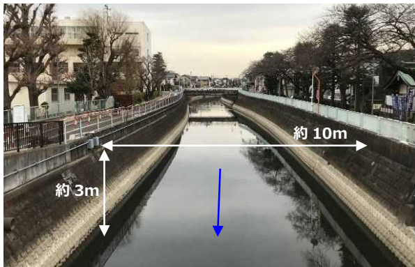
Fig. 7 Field situation (upstream from Tekona Bridge)
