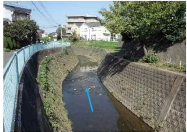
Fig. 1 A urban river covered with concrete revetment
