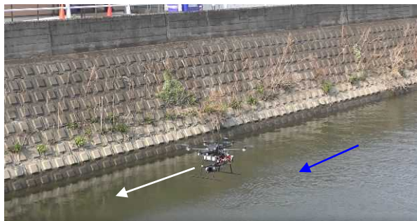
Fig. 8 Flight situation (around Sugano Bridge)
