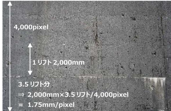
Fig.5 The Accuracy verification of photography image
