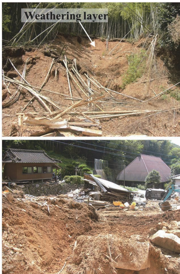
Fig.11 Collapse (upper) and damage (lower) in Fushiki, Ashikita Town (photos taken on August 1, 2020)
