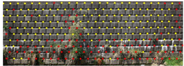
Fig. 1 Block coordinate (yellow points) detected by template matching and block coordinate (red points) obtained by interpolation
