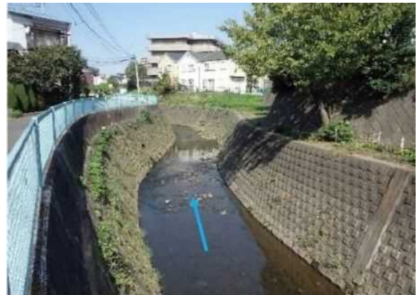
Fig. 1 A urban river covered with concrete revetment
