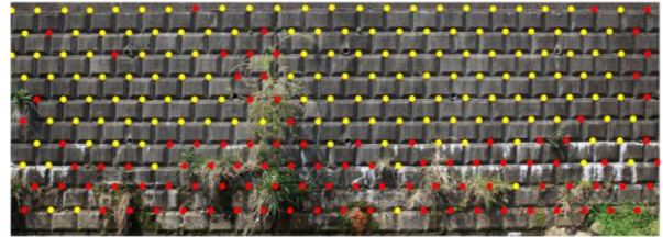
Fig. 1 Block coordinate (yellow points) detected by template matching and block coordinate (red points) obtained by interpolation
